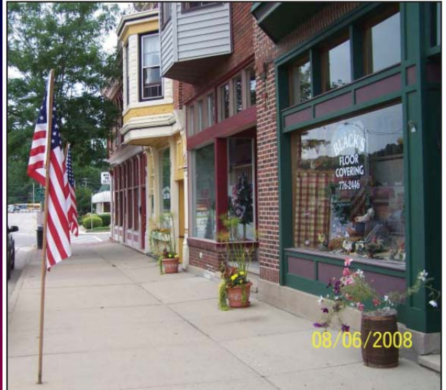
Historic buildings that grace Darlington's Main Street are protected from flood damage and their historical character is preserved. Photo: Barbara Ellis, FEMA
