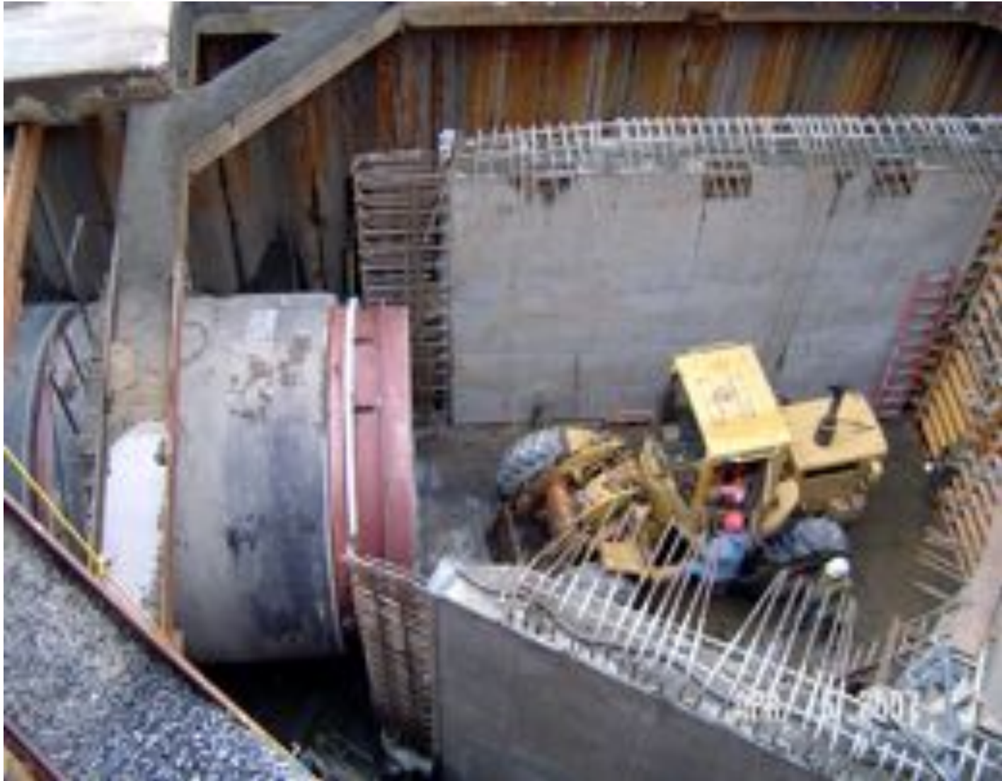
Large diameter conveyance pipeline dwarfs front end loader and operator
