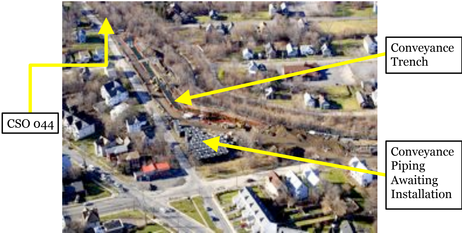
Conveyance project under construction through south side neighborhood causing significant disruption
