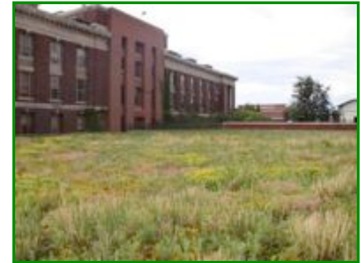
Green Roof at SUNY ESF
