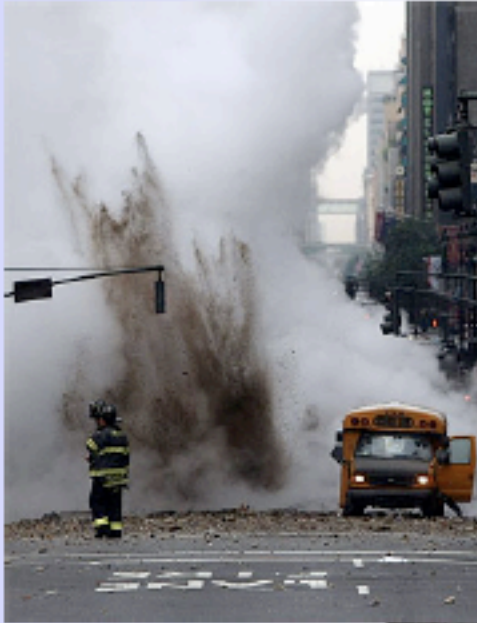
NYC pipe explosion, July 2007 Credit: Mario Tama, Getty Images
