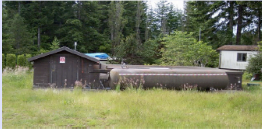
Small system wellhead with hydrotank Credit: Rural Community Assistance Corporation
