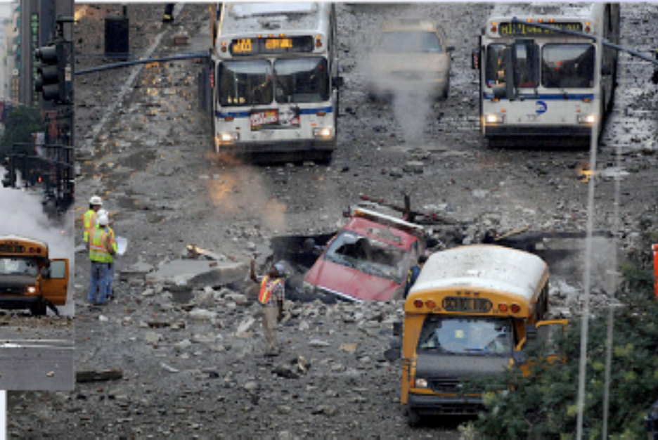
NYC pipe explosion, July 2007 Credit: Robert Stolank, New York Times
