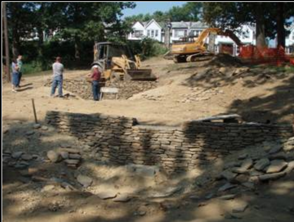
Garden Walls Under Construction
