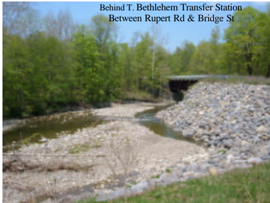
Site of significant erosion
