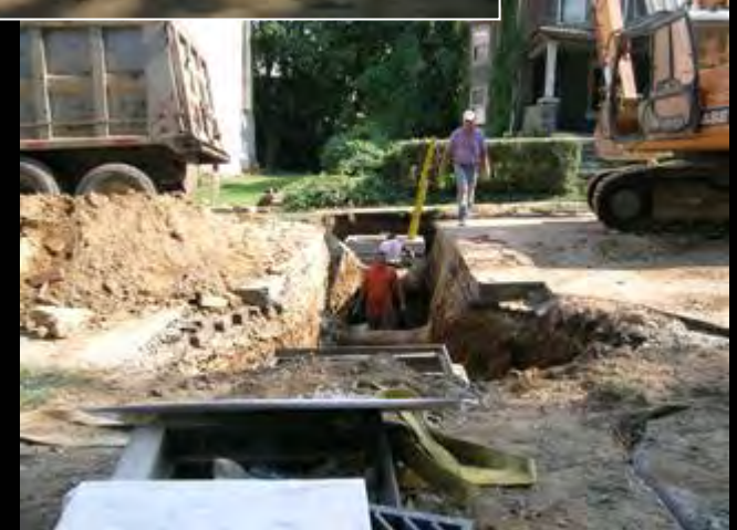
New Inlets to Divert Street Runoff
