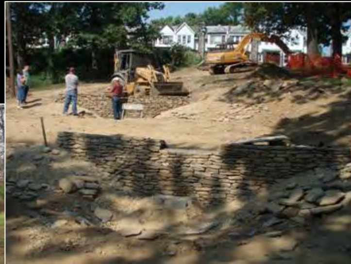
Garden Walls Under Construction
