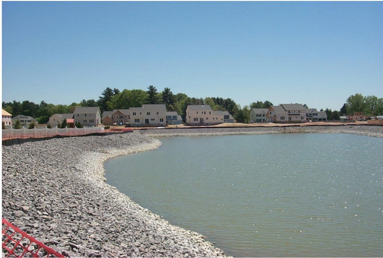
Large stormwater retention basin for new housing development in Guilderland.
