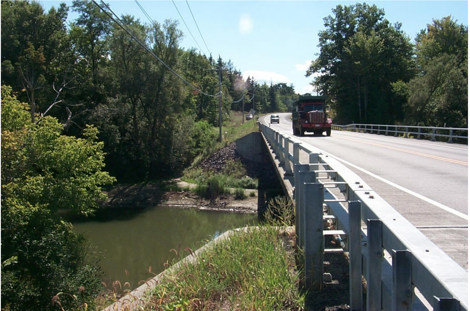
State Highway 158 crossing the Normans Kill at the reservoir inlet.
