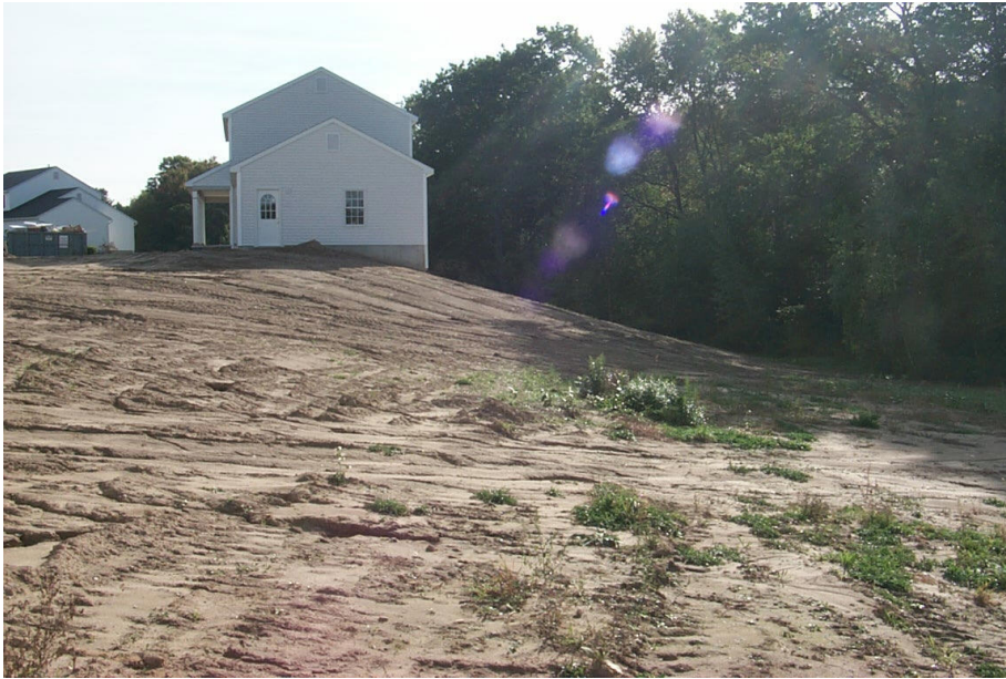
Erosion from a housing development in Rotterdam heading toward a Normans Kill tributary.
