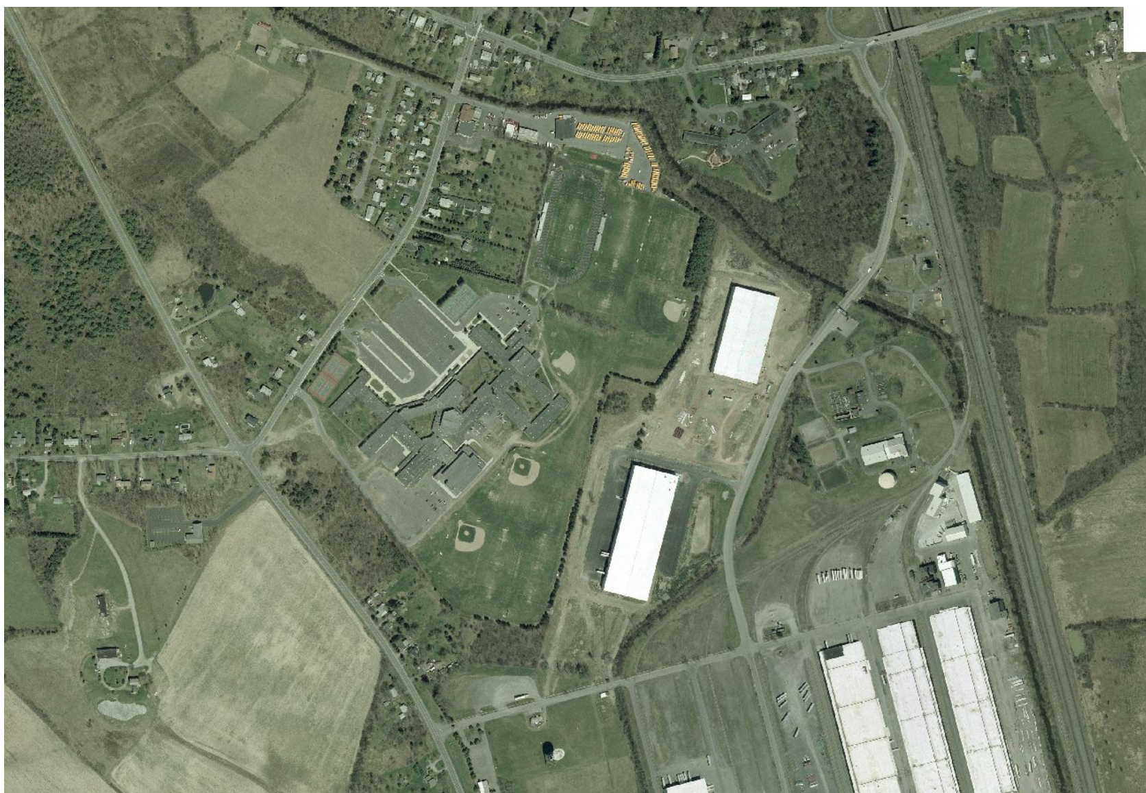
Location of migrating toxic groundwater plume from Northeast Industrial Park superfund site heading toward Guilderland High School. Bus Garage at top next to Black Creek.
