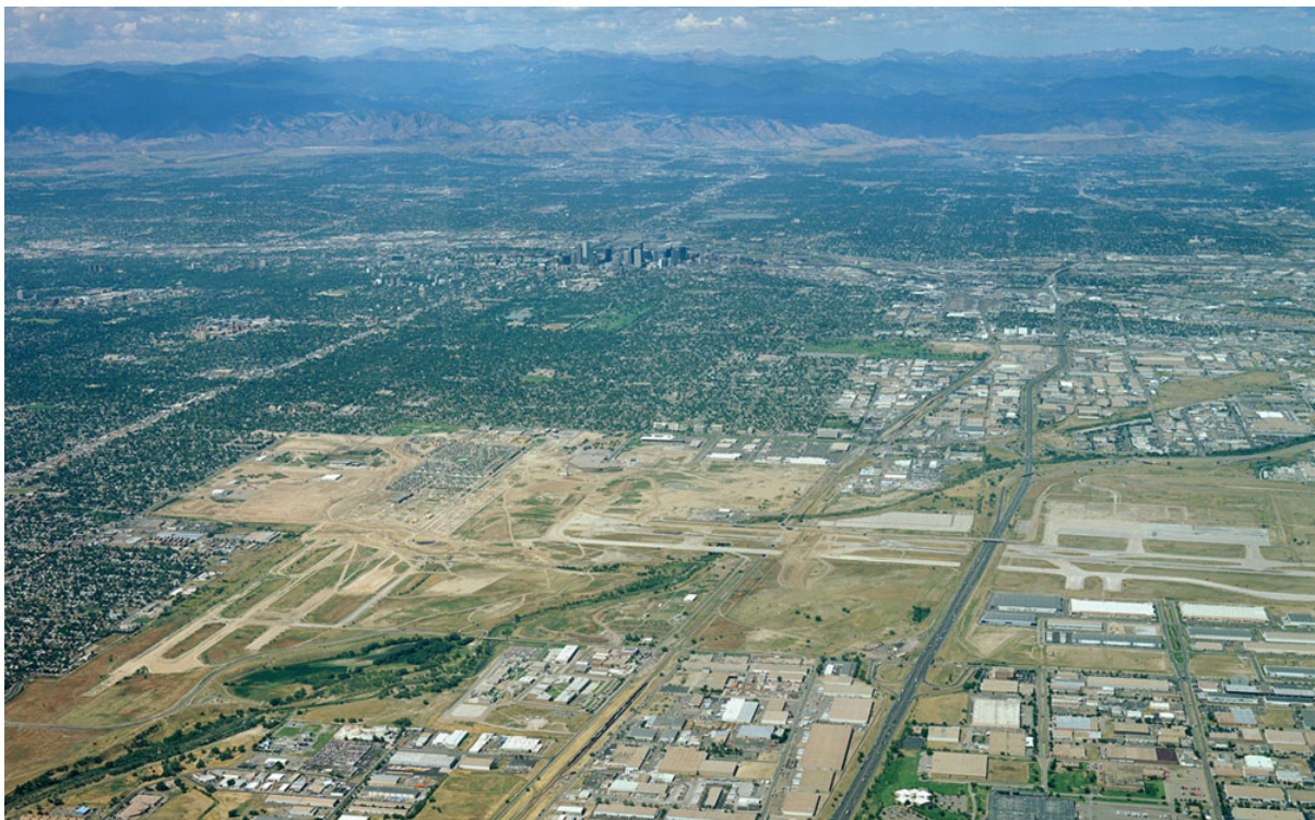
Figure 5.6 Stapleton Site at the Start of Construction
