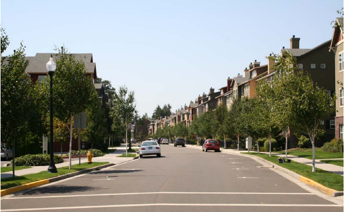
Figure 5.29 Garden Apartments at Orenco Station South
