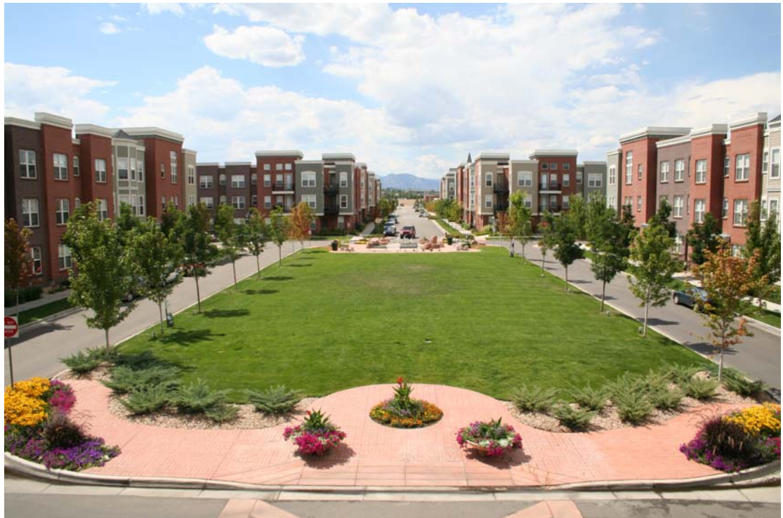
Figure 5.5 Bradburn Apartments and Village Green
