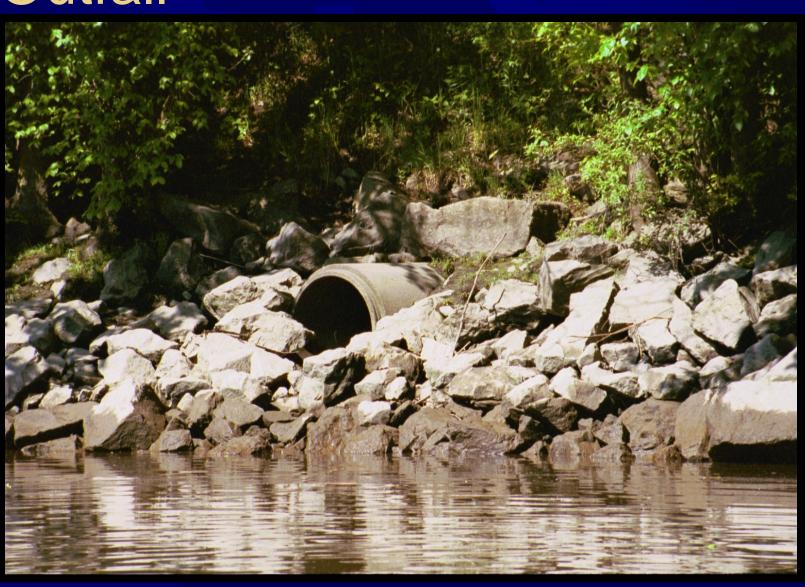
Combined sewer systems are designed to discharge directly to surface waterbodies such as rivers, estuaries, and coastal waters during wet weather, when total flows exceed the capacity of the CSS or treatment plant.
