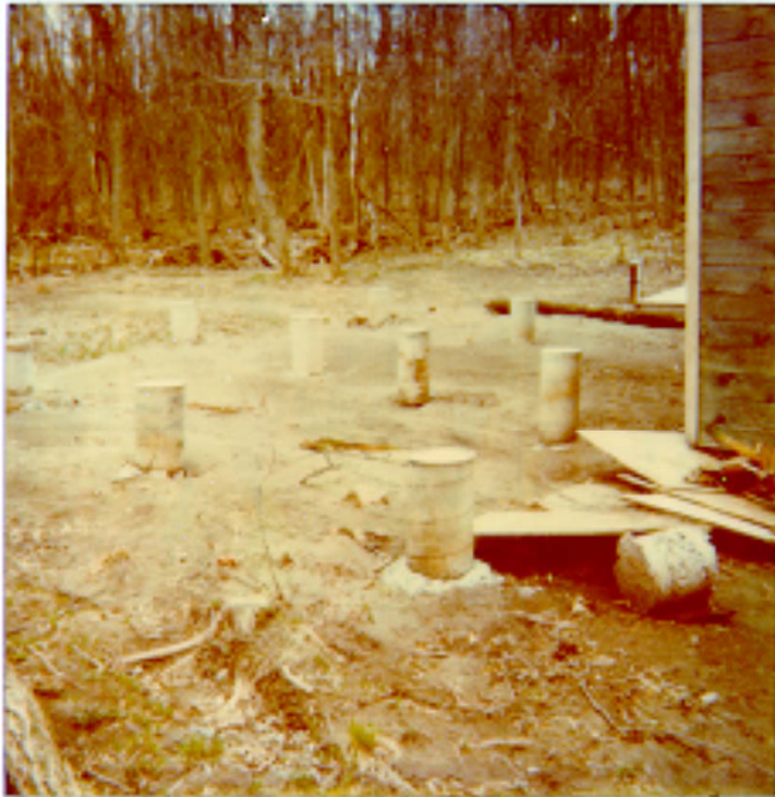
(T) Charleston - End of Butler Dr - adjacent to creek - additional photo 4/24/96
