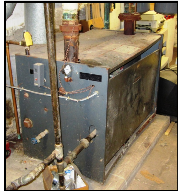
Visitor's Center, Saratoga Springs
