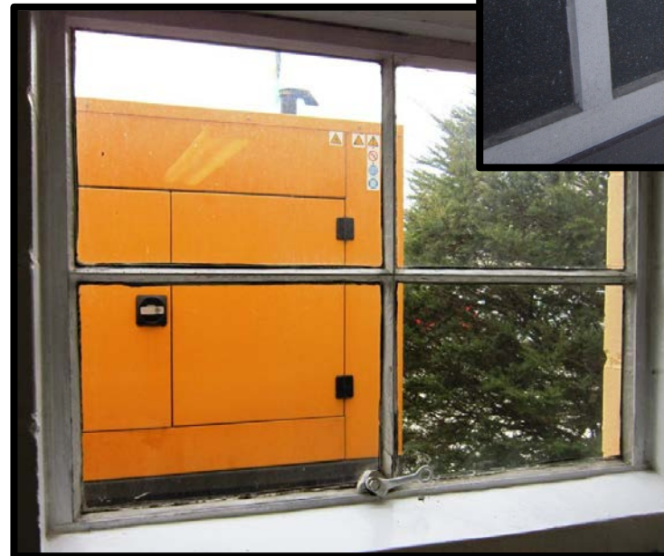
Highway Garage, Clifton Park
